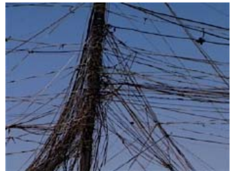
Tapping into the grid is something done throughout Iraq. Here, several dozen households attempt to sap a bit of power, which only blows a transformer and sends residents to another tower. This wire situation is not uncommon, but military vehicles also can complicate matters by unintentionally ripping down low-hanging cables with their high reaching antennas.
