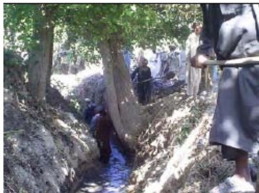
Work on a section of the Deh Mian Karez
